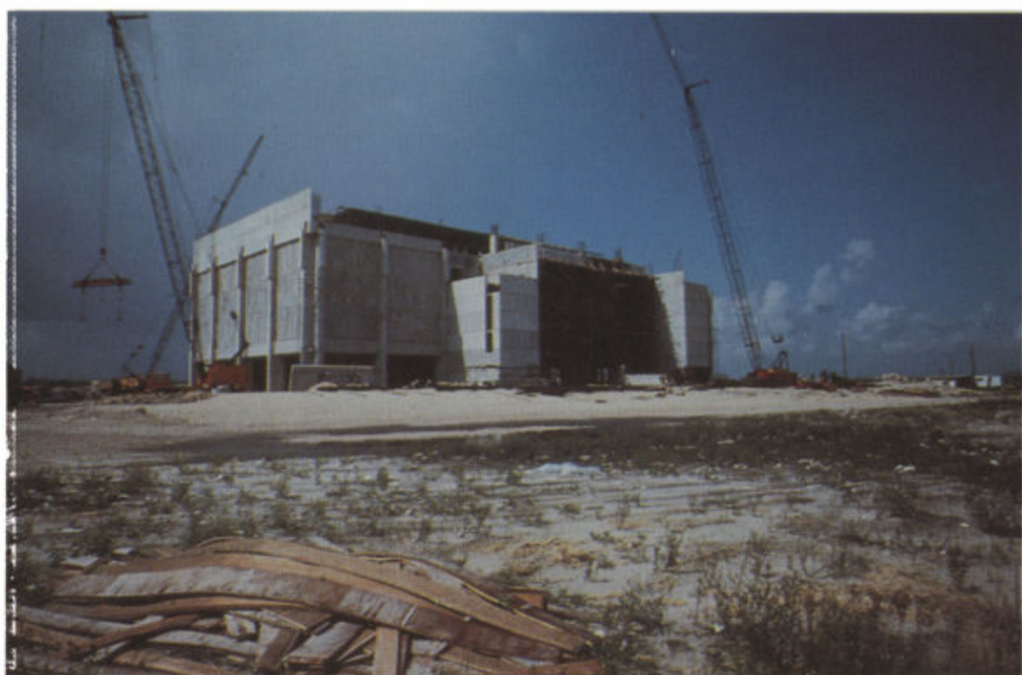
Construction for Primera Casa, the University's first major building.
